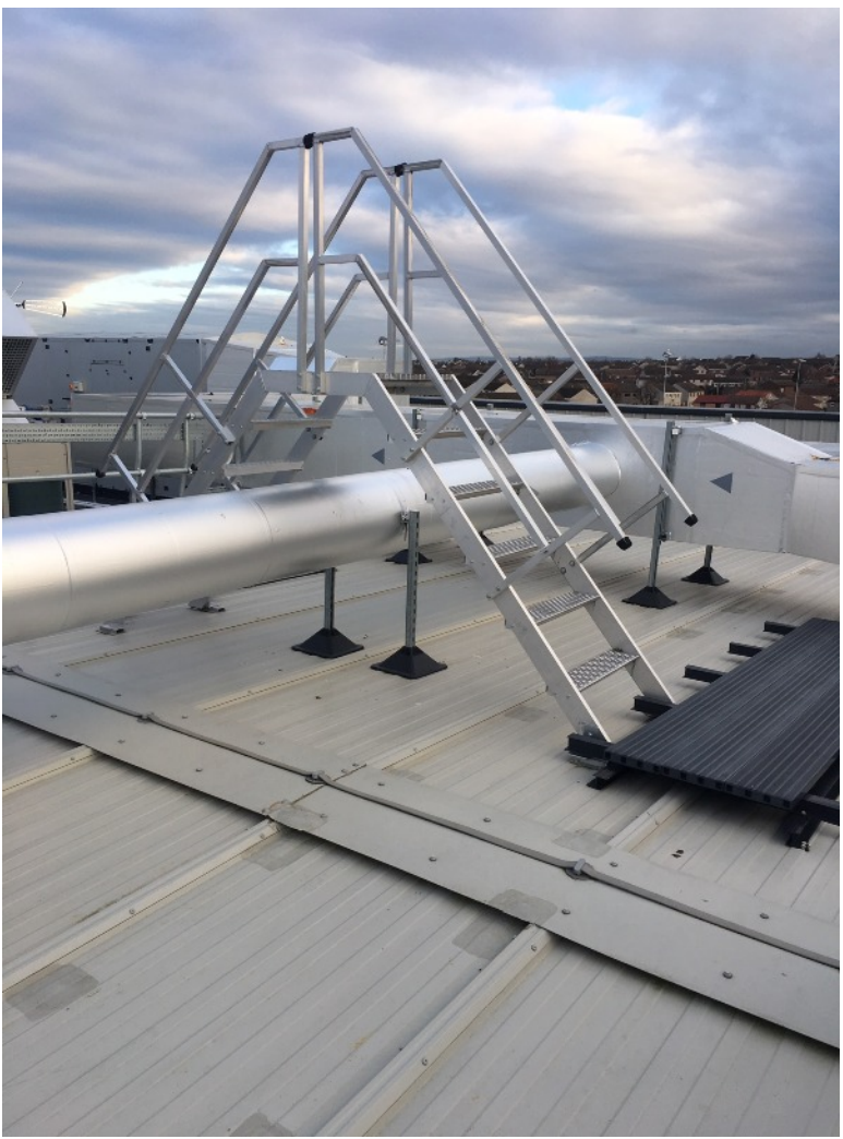
A sample of Crossover Ladders supplied and installed by our engineers.
